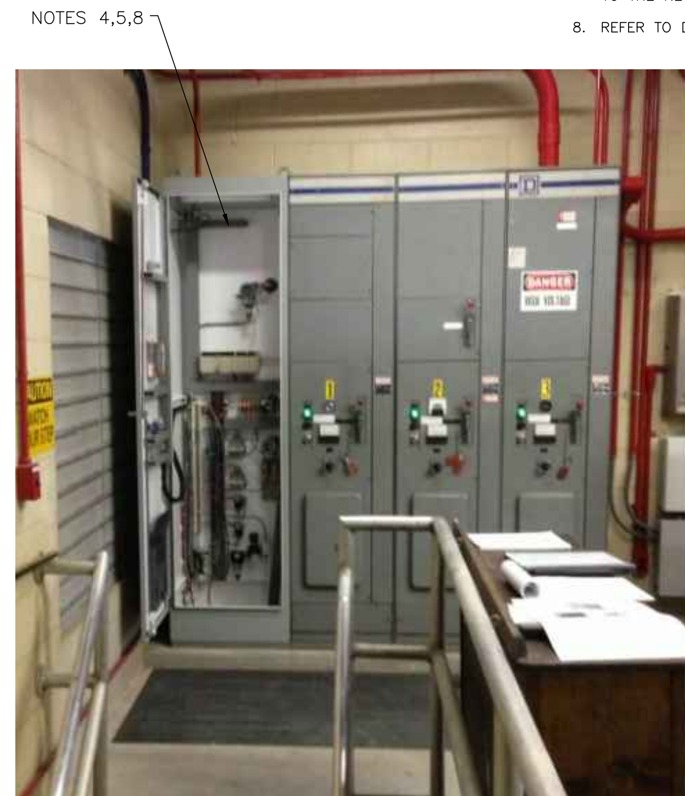
4 EXISTING CONTROL PANEL SCALE: NOT TO SCALE
