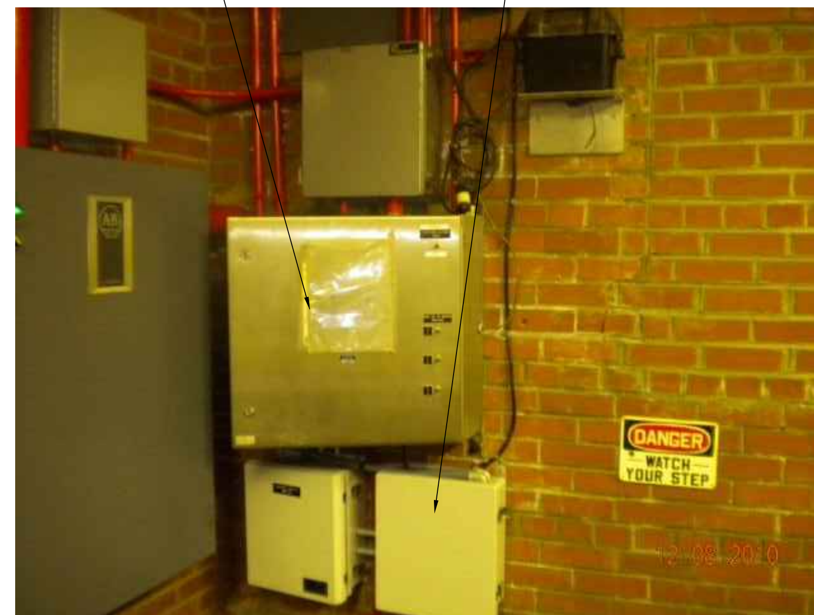
3 EXISTING MOSCAD PANEL SCALE: NOT TO SCALE
