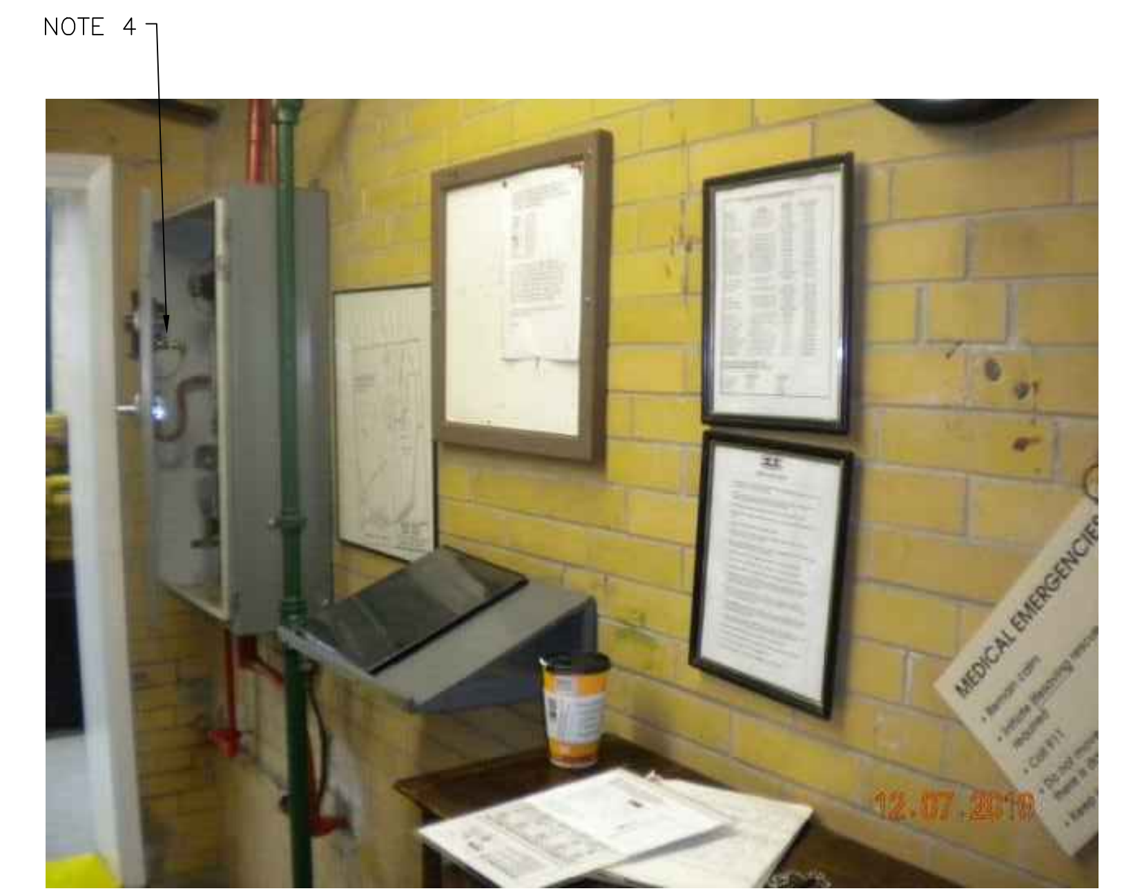
4 EXISTING CONTROL PANEL SCALE: NOT TO SCALE
