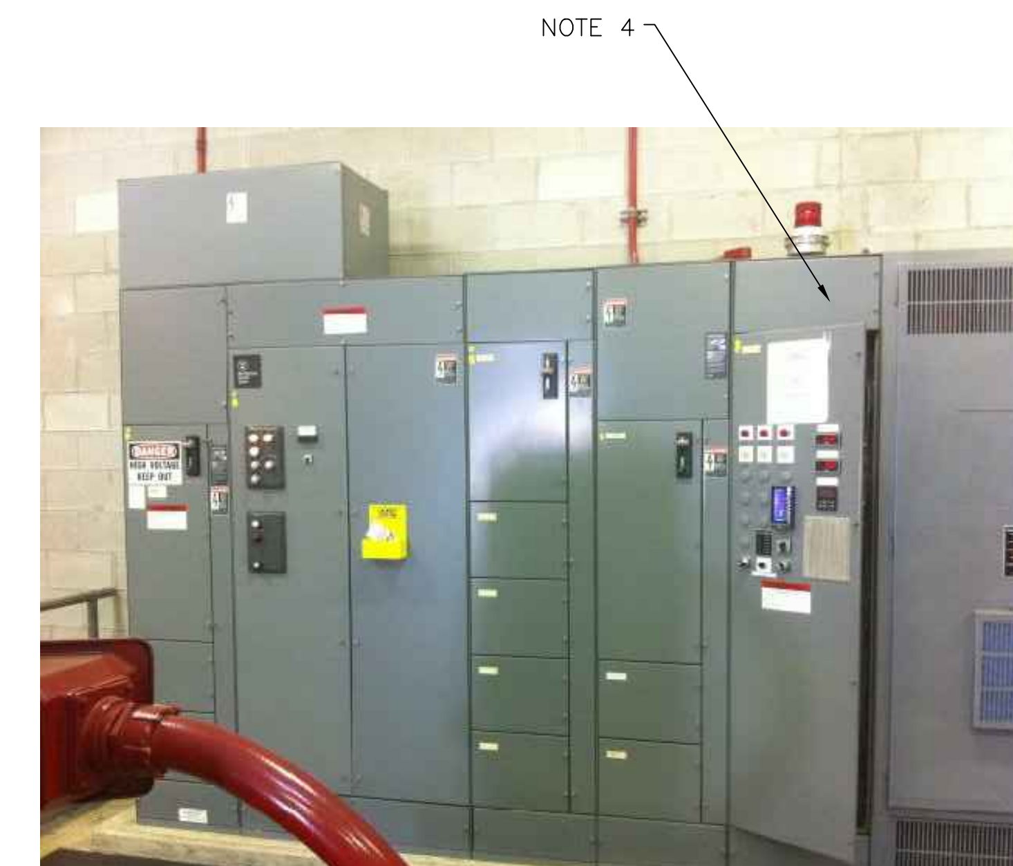
4 EXISTING CONTROL PANEL SCALE: NOT TO SCALE
