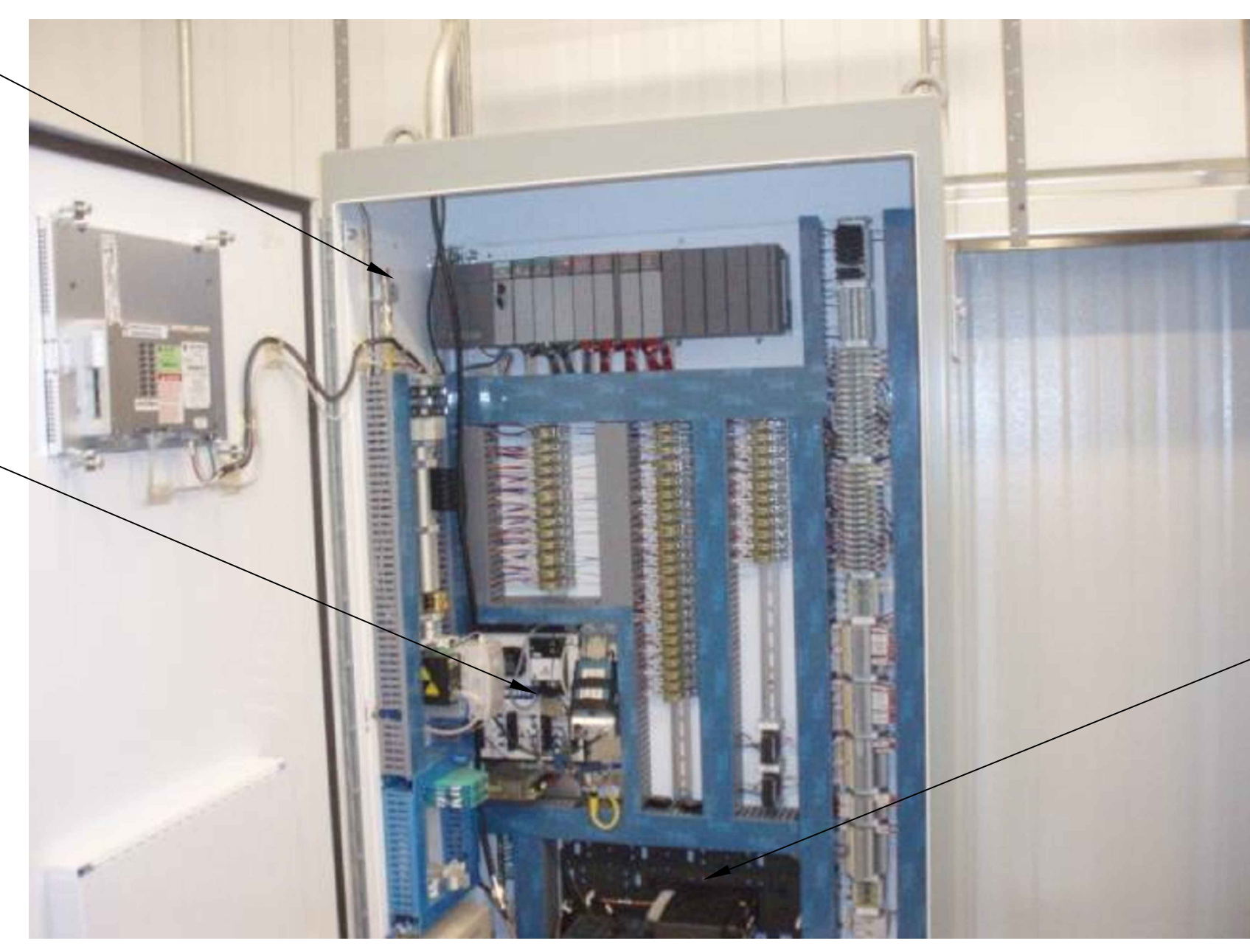
3 EXISTING CONTROL PANEL SCALE: NOT TO SCALE
