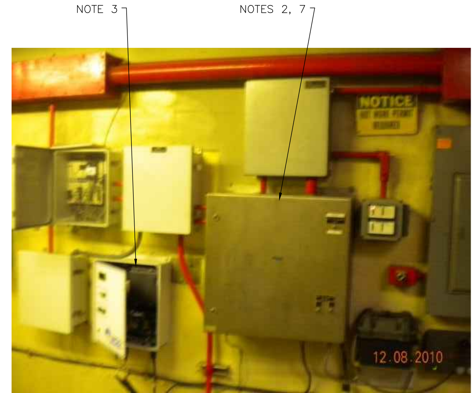
3 EXISTING MOSCAD PANEL SCALE: NOT TO SCALE
