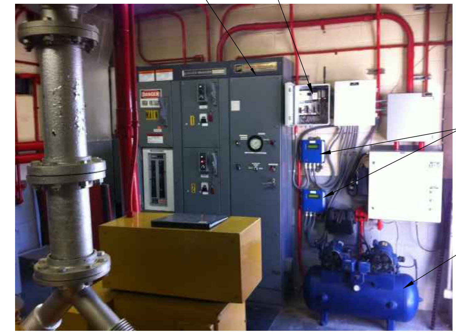
4 EXISTING CONTROL PANEL SCALE: NOT TO SCALE
