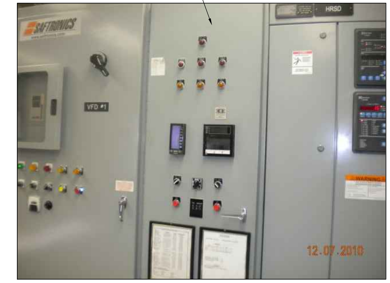
4 EXISTING CONTROL PANEL SCALE: NOT TO SCALE
