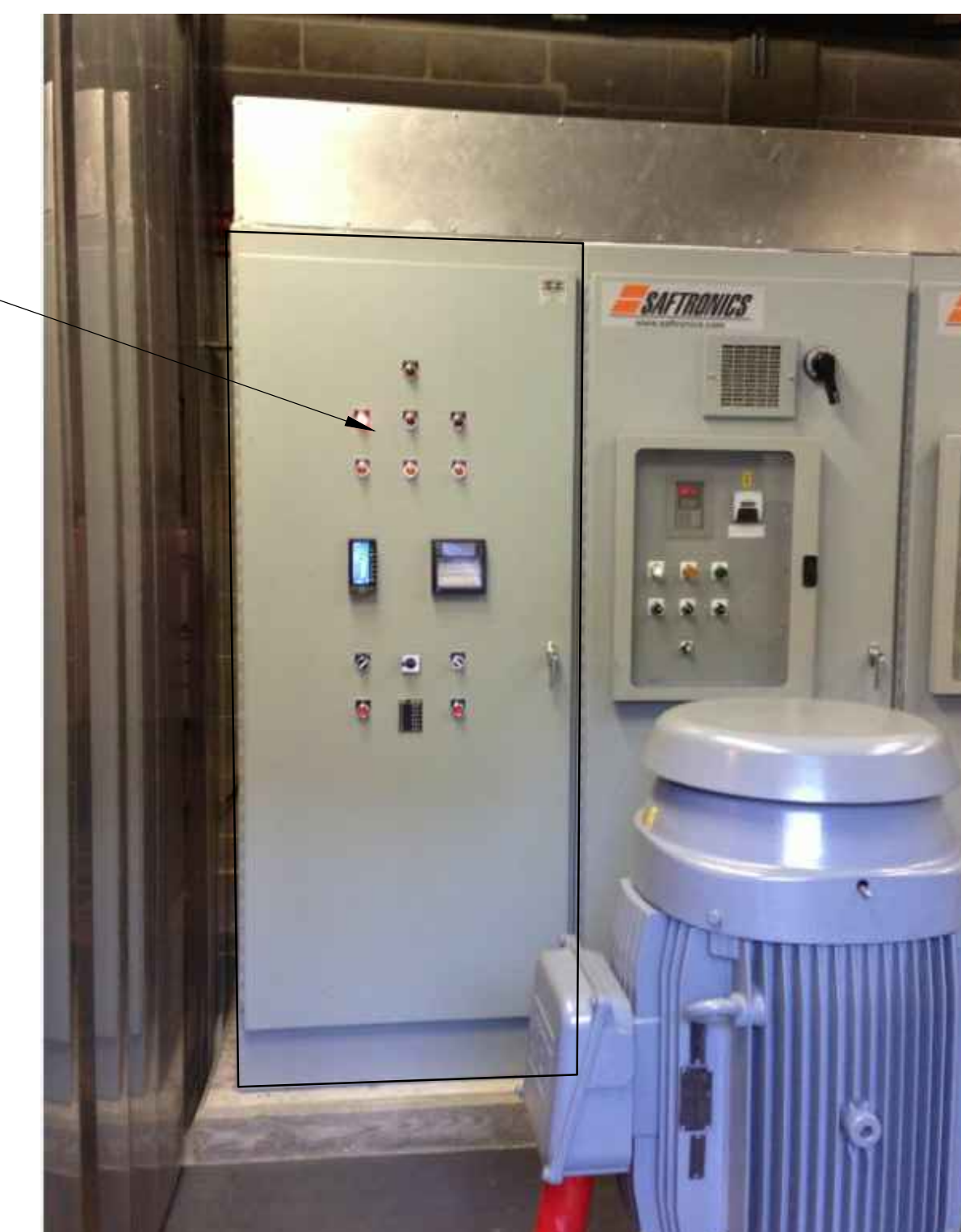
4 EXISTING CONTROL PANEL SCALE: NOT TO SCALE
