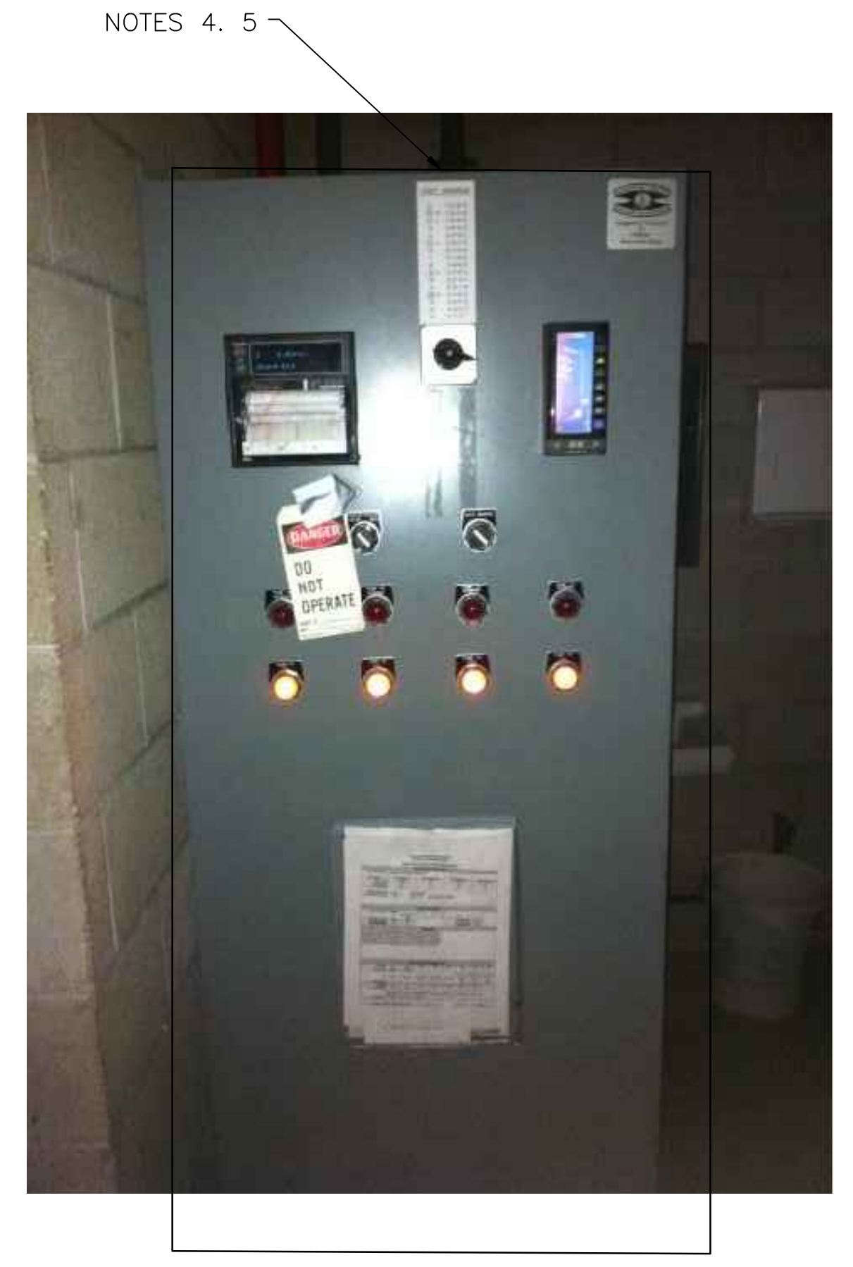
4 EXISTING CONTROL PANEL SCALE: NOT TO SCALE
