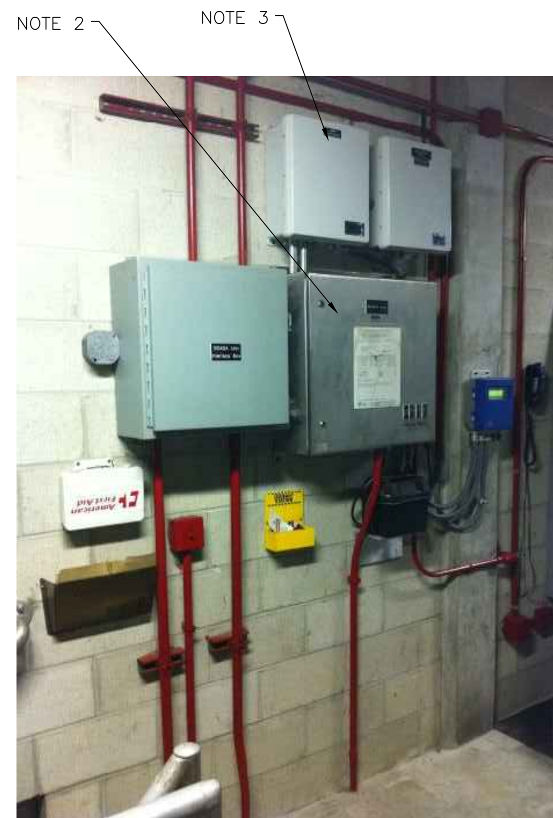
3 EXISTING MOSCAD PANEL SCALE: NOT TO SCALE
