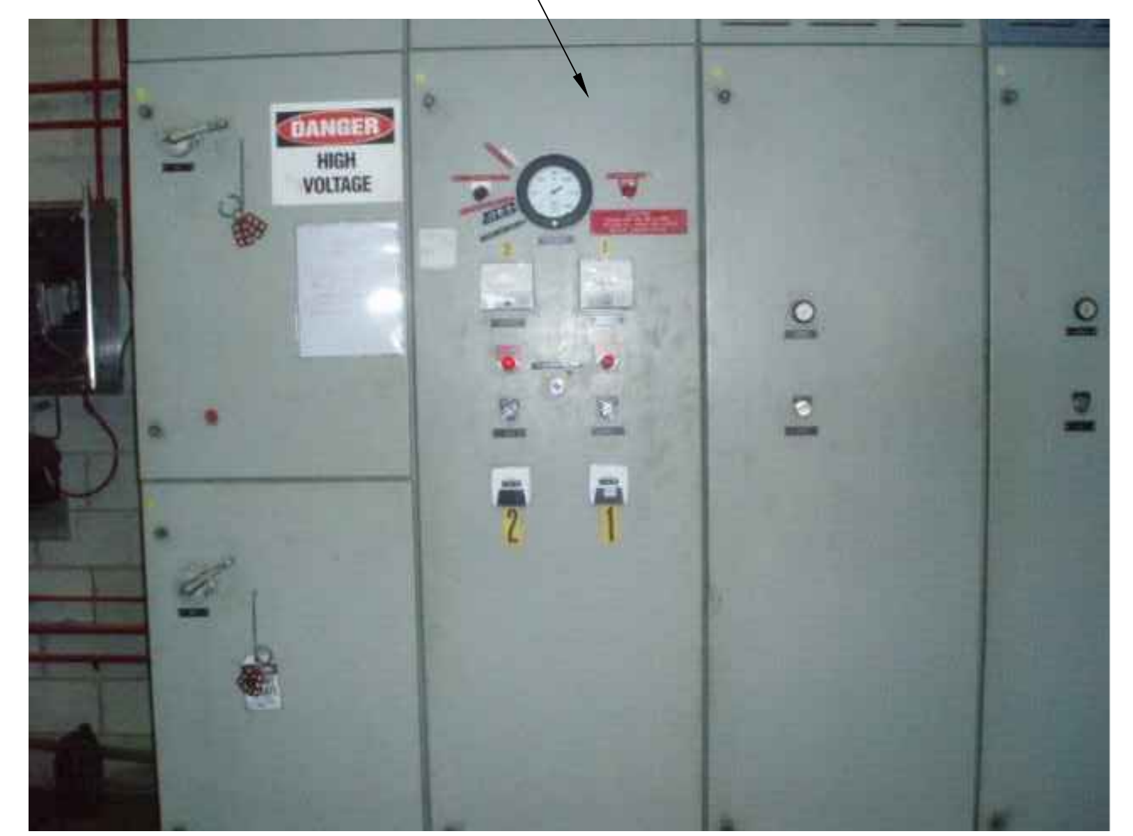
3 EXISTING CONTROL PANEL SCALE: NOT TO SCALE
