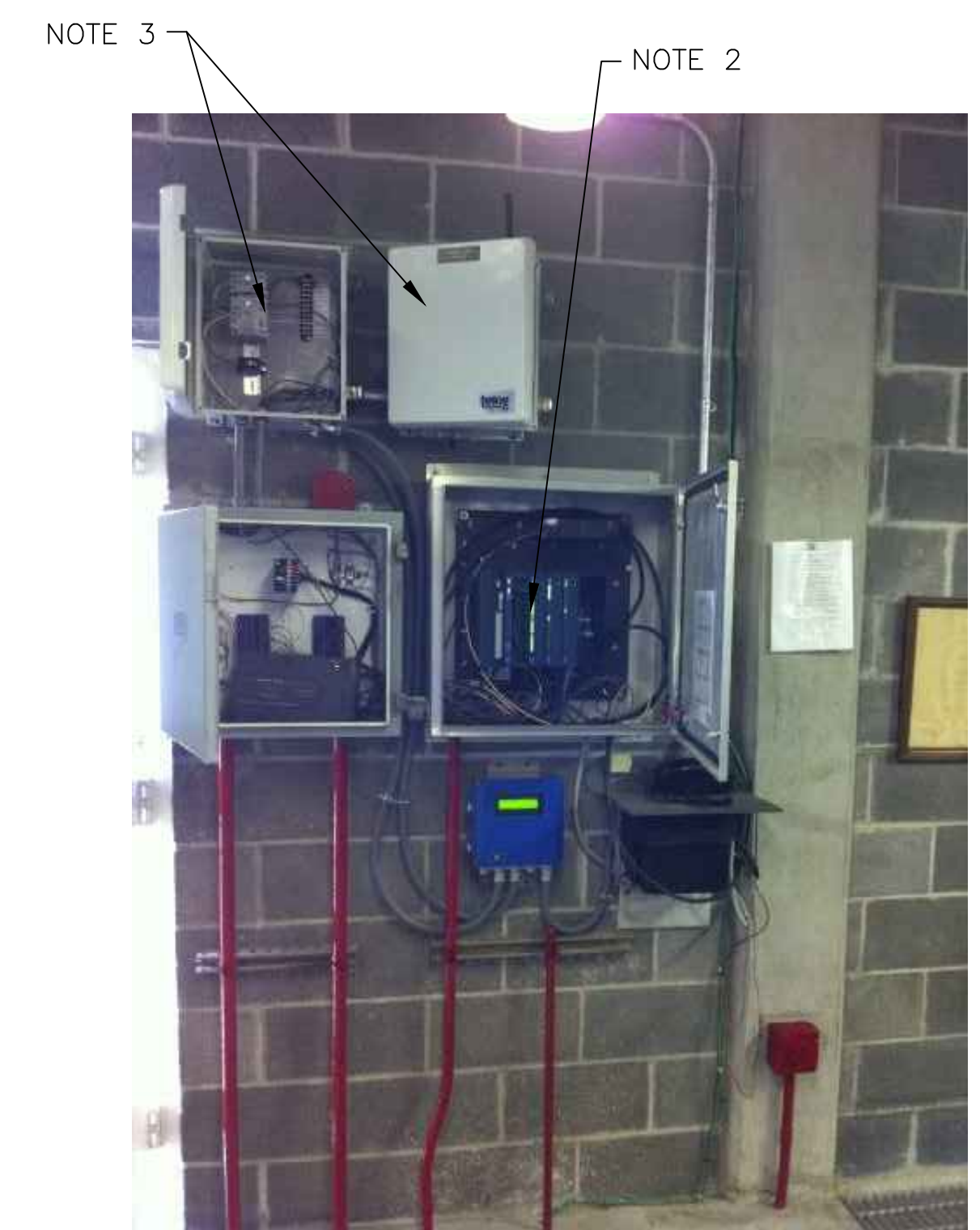
3 EXISTING MOSCAD PANEL SCALE: NOT TO SCALE
