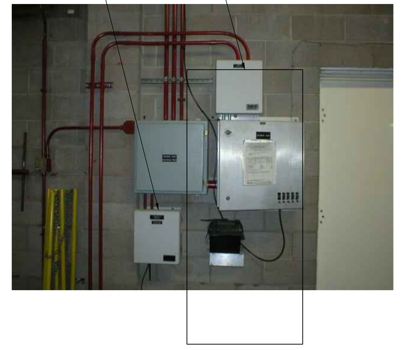
4 EXISTING MOSCAD PANEL LOCATION SCALE: NOT TO SCALE
